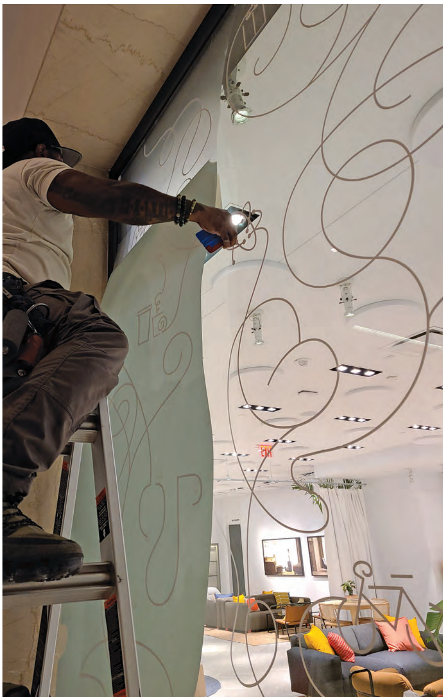
Example of a larger CAD-cut vinyl job utilizing registration blocks on the top for proper alignment of the panels.
