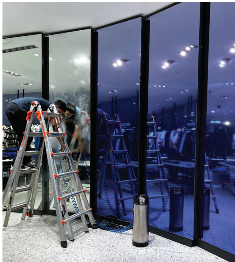
Solvent ink transparent graphics being applied to mirrors. The mirror could not be seen if we produced these graphics on our UV printer.
