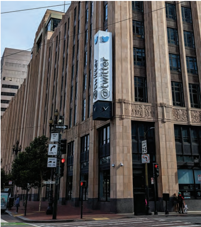
Colite produced the Twitter blade sign in downtown San Francisco. This iconic three-sided behemoth was an architectural blade sign marvel with halo-lit lettering and logo complete with functional clocks.
