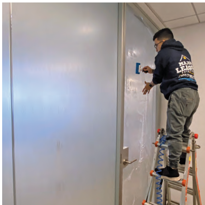
An example of first-surface vinyl applied to glass.
