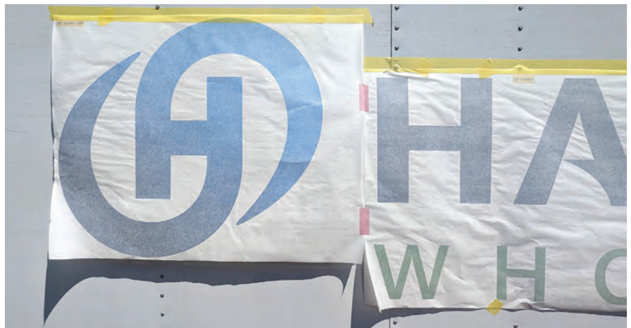
Adding simple alignment blocks speeds up the installation of spot graphics.
