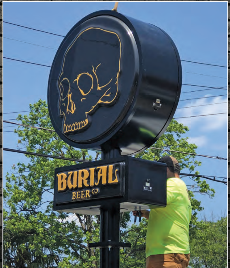
Flynn sets and tightens mounting hardware while checking LEDs.
