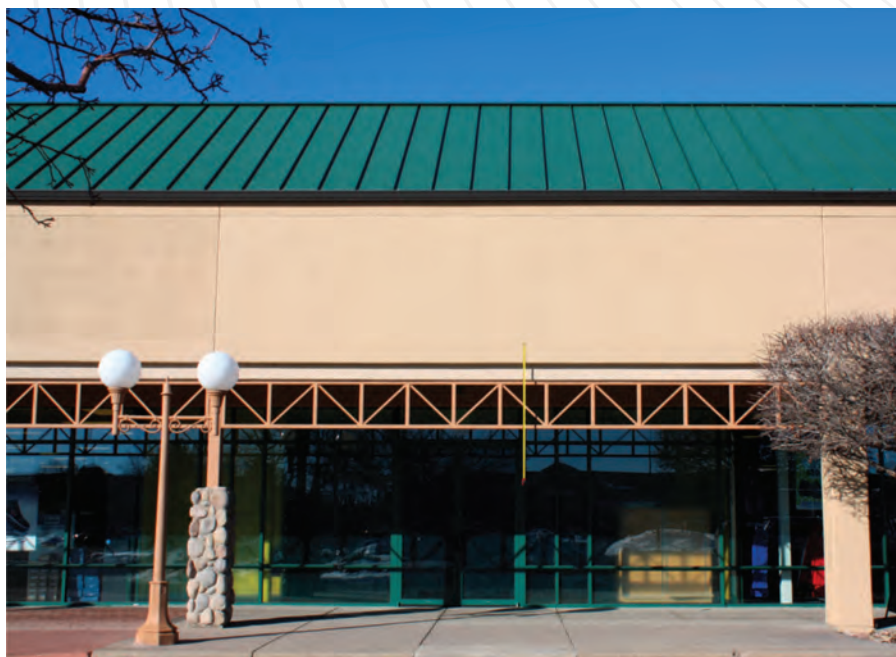
The pre-sale sign survey is critical to obtaining a plethora of data. Taking time to capture straight-on photos is important for providing a clear, focused image for the sign designer to use on the drawing.
