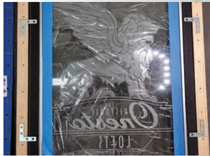
Add angle brackets to the frame to secure glass and anodized channels to the frame.
