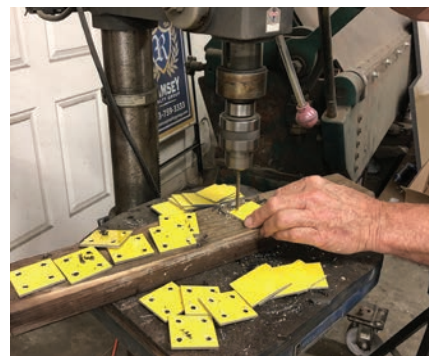
Each pad is drilled with extra holes to give the glue (which will hold them in place) more to bond to.
