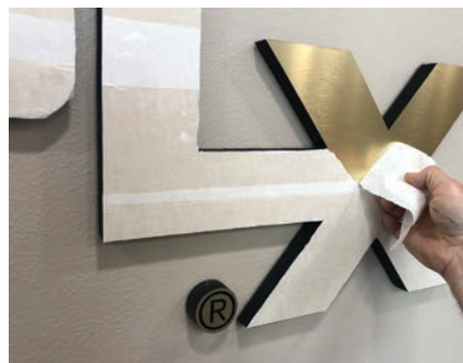
The final step is removing the transfer tape protective sheet, making sure the finish is perfectly clean.
