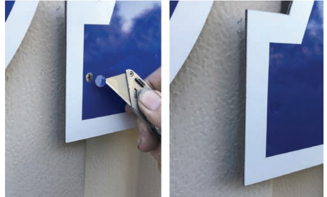
Here our little colored dots come in handy and work well for hiding fasteners.
