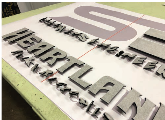
A pattern was printed on paper and then parts were set over the pattern accurately pressed into place, creating an accurate hole pattern for the install.
